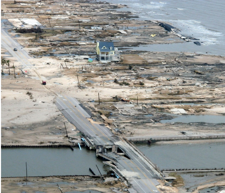
Figure 125: Lone house survives Hurricane Ike. It is reported that this house was rebuilt to withstand a Category 5 hurricane after it was destroyed previously by Hurricane Rita in 2005. 127
