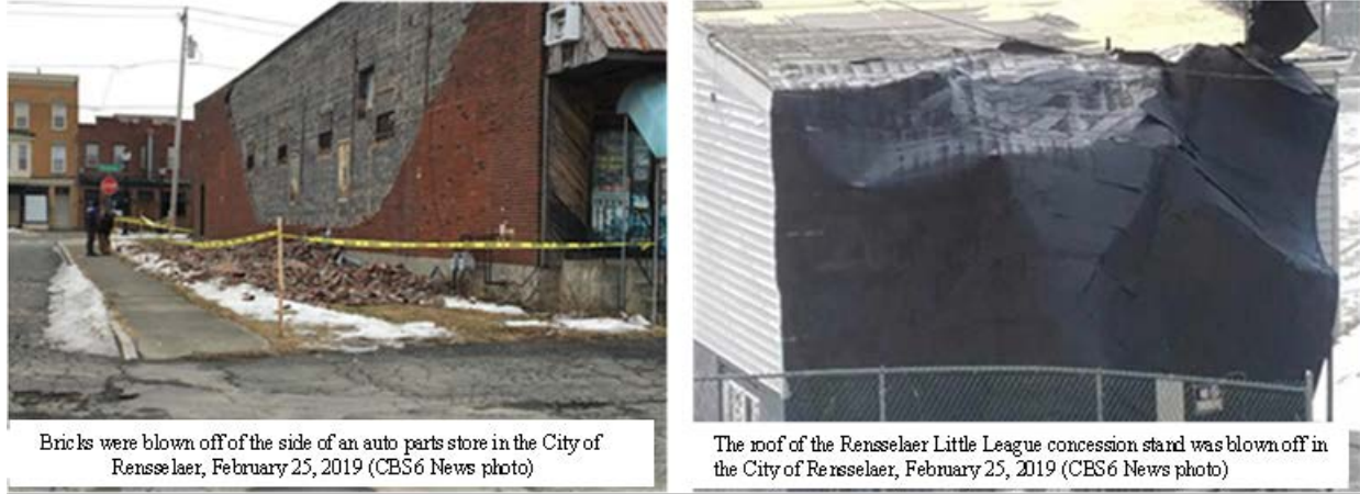
Figure 1: Previous Damage in the City of Rensselaer
